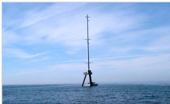
Cape Wind Meteorological Tower Sole operating offshore wind energy met tower in United States
